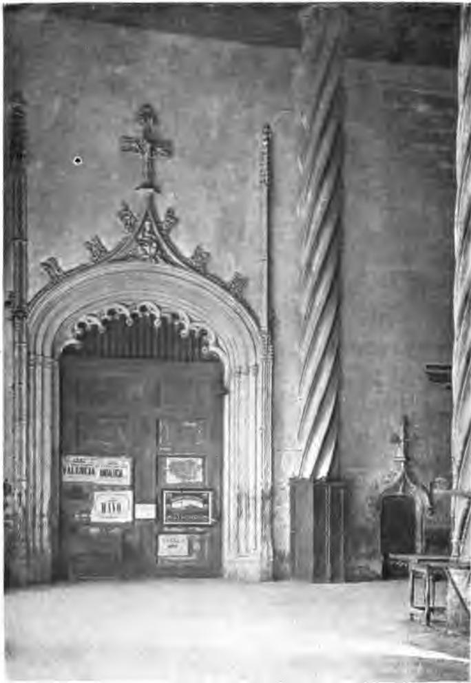
VALENCIA: INTERIOR DOOR OF THE EXCHANGE
